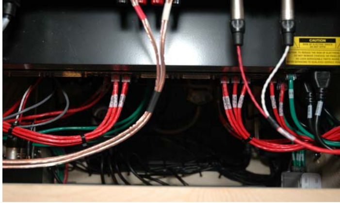
Audio I/O at the Blade are laced and properly labeled
